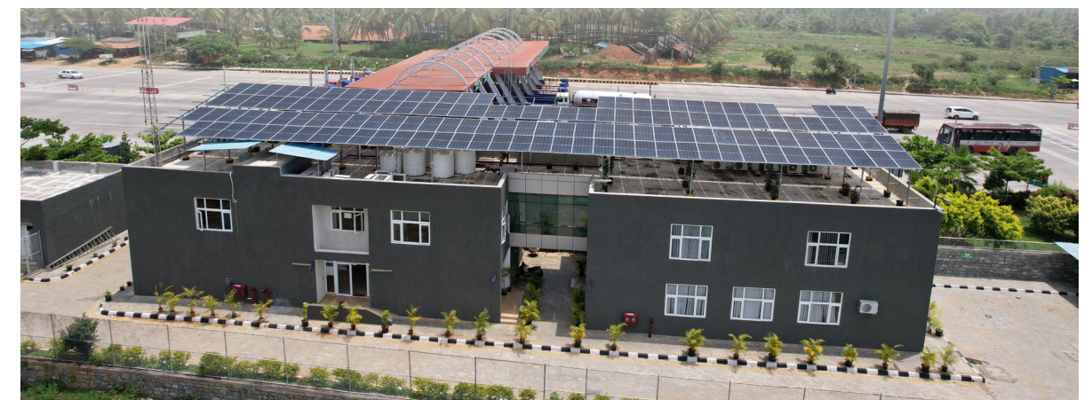
Solar Energy used at Devihalli Hassan Tollway Private Limited
